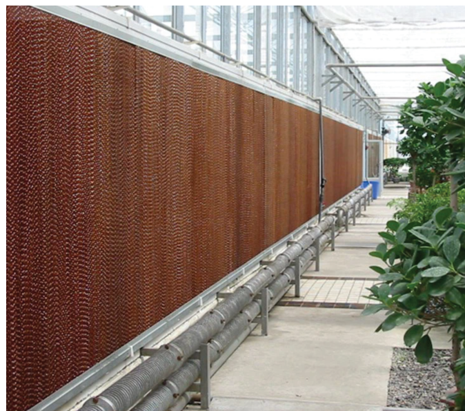
Figure 6.10 Evaporative cooling pad system
